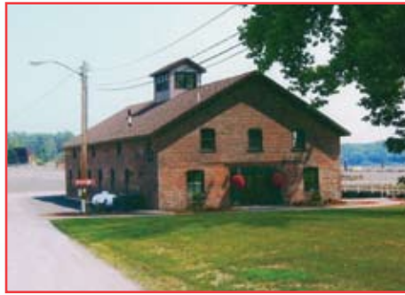
P&M Brick's old horse barn was renovated and now serves as the Port's office.
