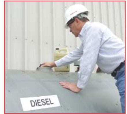
Treat fuel with an additive to prevent bacterial/fungal growth.
