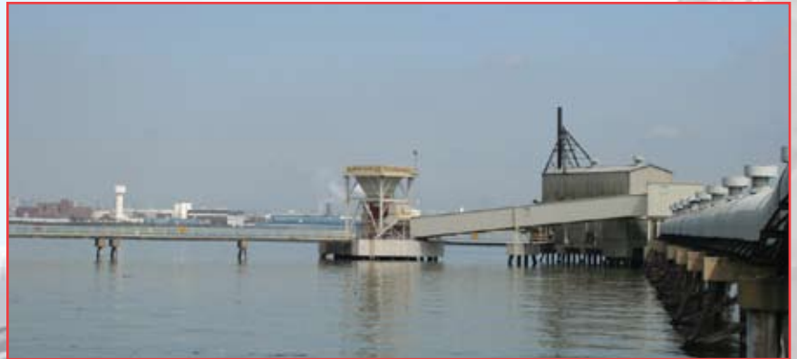
Raw gypsum arrives in rock form on a company ship and is off loaded via conveyor belt.
